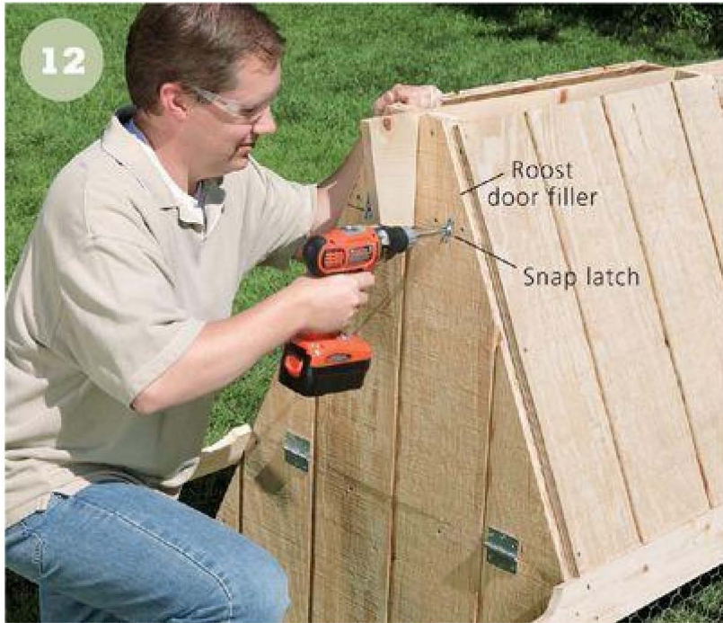
12 Install the end wall and the hinged roost door. The wall is affixed permanently with screws or staples. The door should be hinged from below. Install snap latches to the roost door fillers to secure the door in place when it is raised.
