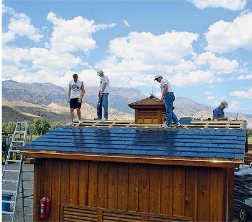
This fiber-cement shingle roof features an integrated array of shingles laminated with thin-film PV modules.
