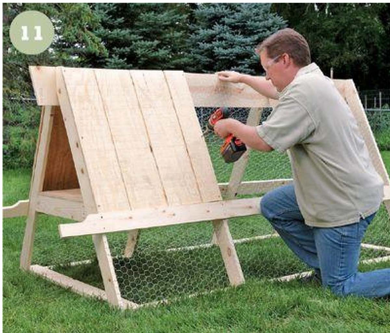
11 Attach the roost side panels to the ark frame with pneumatic nails or staples or with 1-1/4" deck screws.
