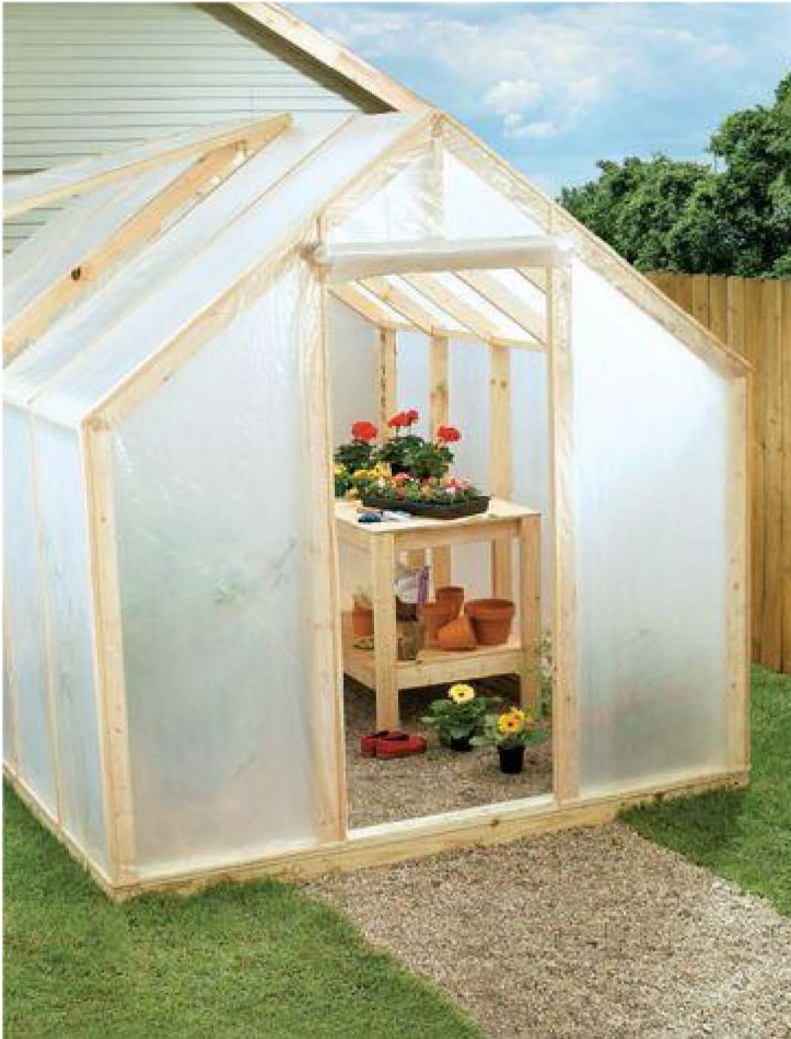
A wood-frame greenhouse with sheet-plastic cover is an inexpensive, semipermanent gardening structure that can be used as a potting area as well as a protective greenhouse.
